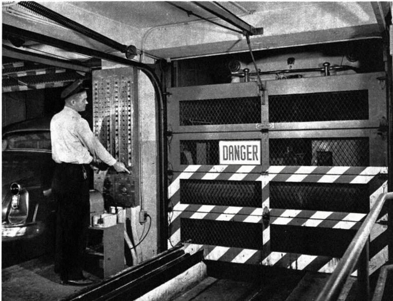
Washington parking facility, completely automatic, is operated from control panel above. Mechanism picks up car, hoists it, parks it. Building is 16 stories high, on narrow lot
